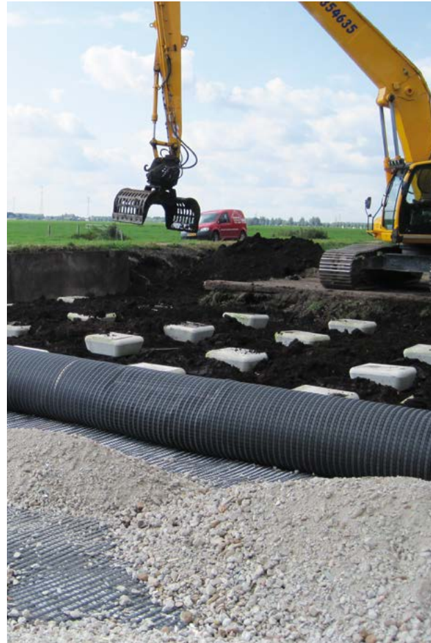
Geotextile reinforcement installed on piles (N 210; Netherlands)
