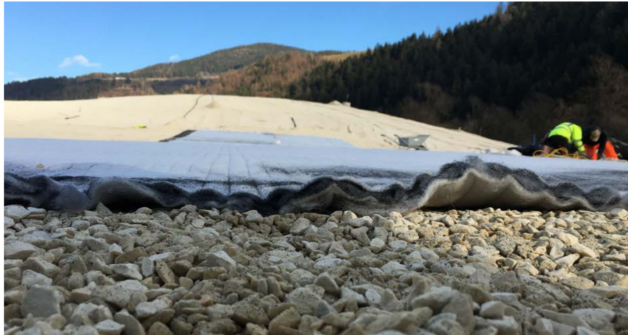
Sealing of contaminated sites
